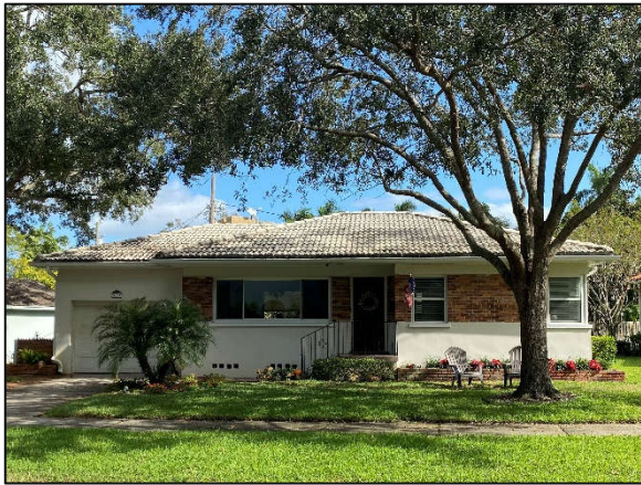
Figure 7: Noncontributing property at 2411 Andalusia Way NE
