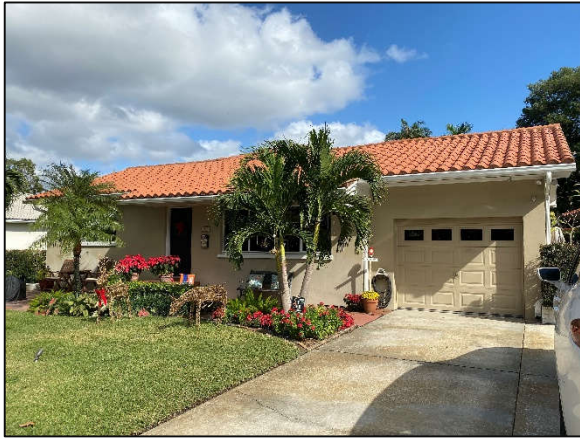
Figure 5: Noncontributing property at 2401 Andalusia Way NE
